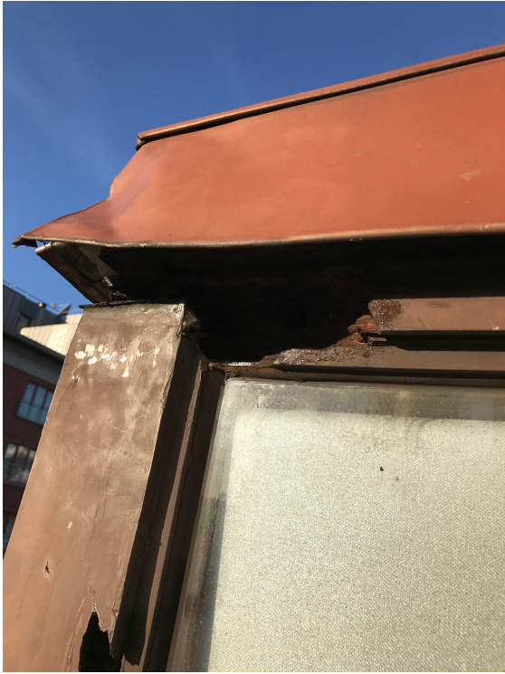
Photos of repairs Jan 2017
